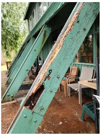
The exposed A frame beams in the dormitories are in need of work. All need to be inspected, some will need to be replaced, and all will be getting a metal sleeve to protect to wood from the elements, as well as provide protection from fire.
